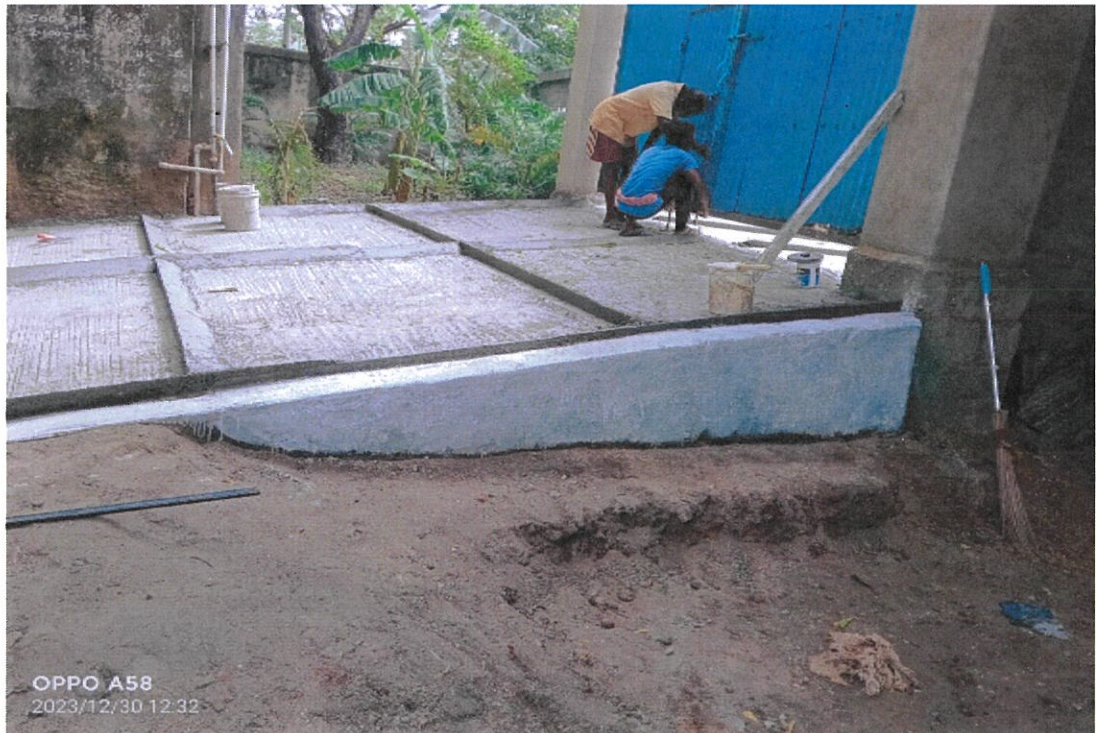
Figure 6 concreting of Ramp completed
