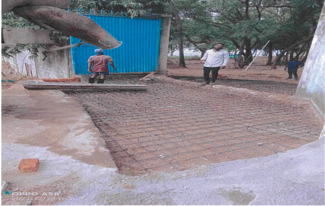
Figure 5 Laying of reinforcement for Ramp
