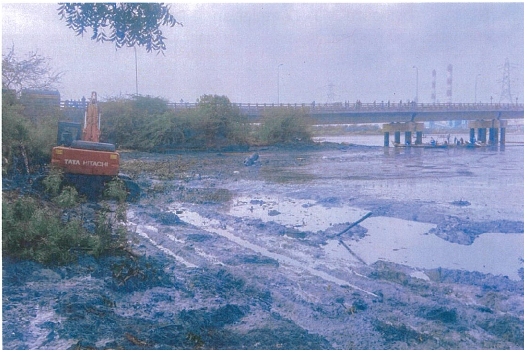
Figure 2 Sludge removal Operation
